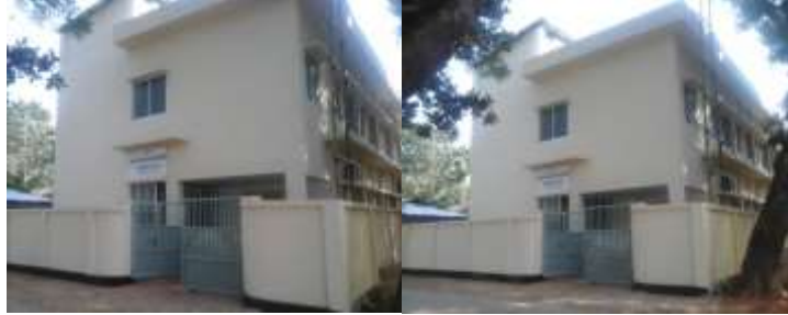
Fig 1 Construction of 1 st floor lab building and boundary wall
